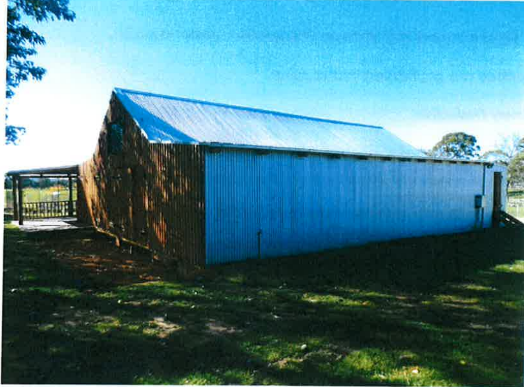
Photo 3: Rear of building proposed to be used as a "Function Centre"
