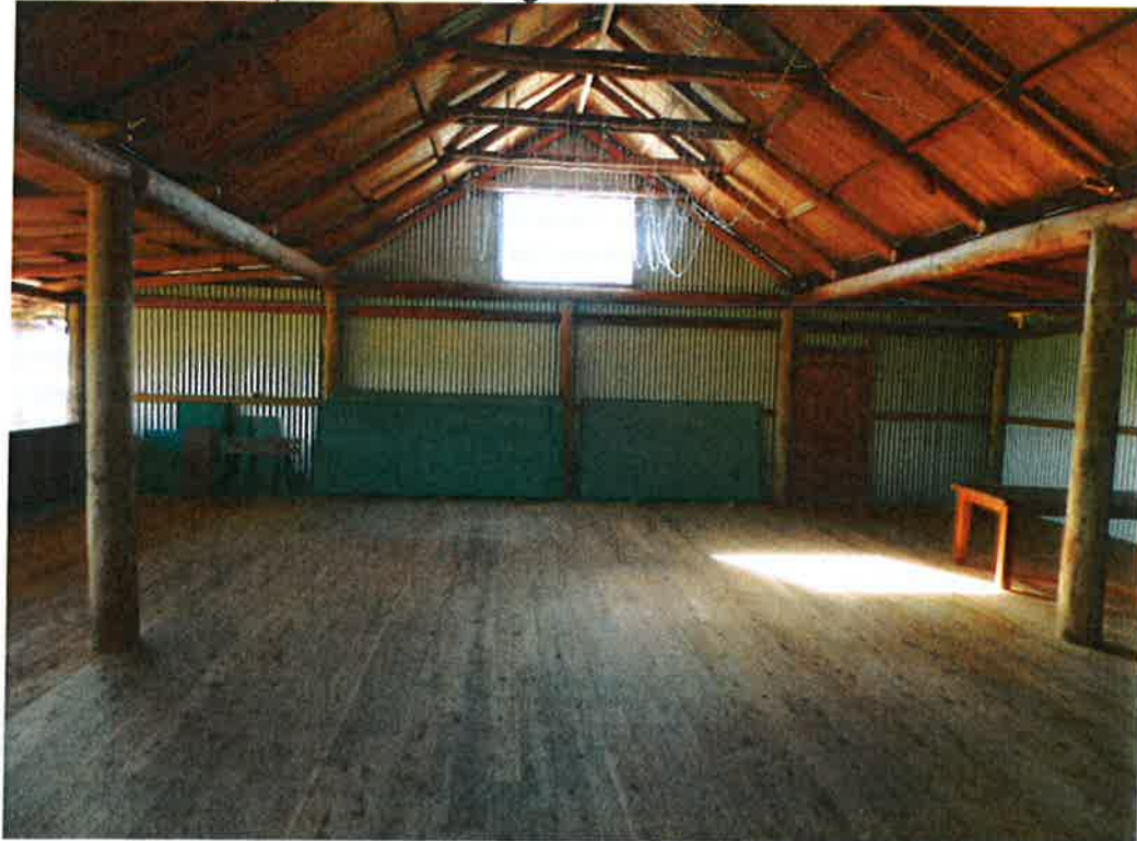
Photo 4: Internal photo of building to be used as a "Function Centre"
